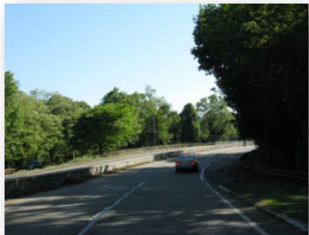
Traveling southbound on the Palisades Interstate Parkway to Fort Lee
