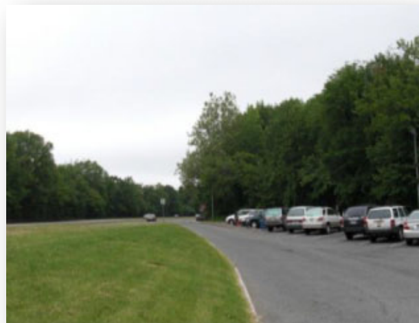
Northbound Service Station, facing north
