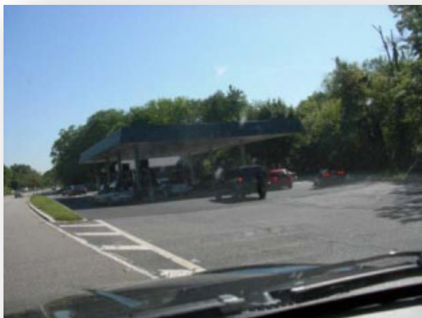
Southbound Service Station, facing south
